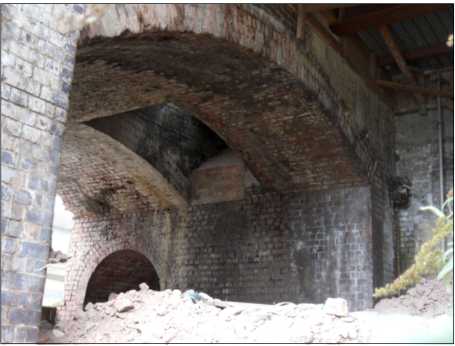
EXISTING PARTIALLY COLLAPSED VAULTS CONNECTED TO LISTED VIADUCT ON BRAITHWAITE ST TO BE REMOVED.
